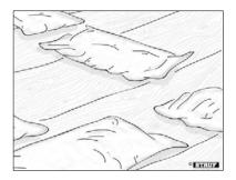
The areas along the edges of the floor and the rows which were installed last are particularly important. The floor should not be used until the glue has cured. Sanding and finishing should not be performed until at least 48 hours after the full-surface gluing.
